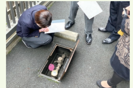
Checking water equipment
