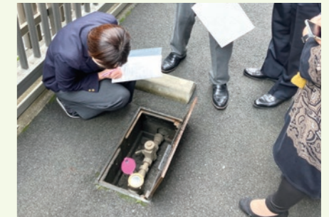
Checking water equipment
